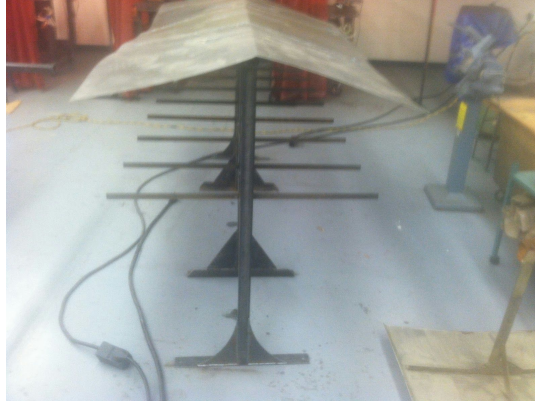
Maverick preparing to weld on the Super ATV gas racks roof.
